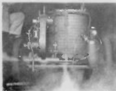
Forced Circulation boiler under test by J. Eggleton.
